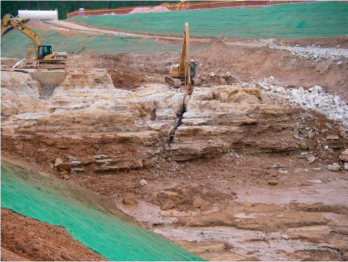
Figure 2. Irregular packstone surface detected in seismic refraction survey.
